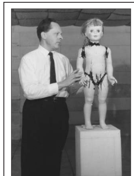
Schwan with model of human body used for RF dosimetric studies. The model is filled with tissue-equivalent liquids and exposed to RF energy in a microwave anechoic chamber that Schwan had constructed in his laboratory. Photograph from ca. 1963.
